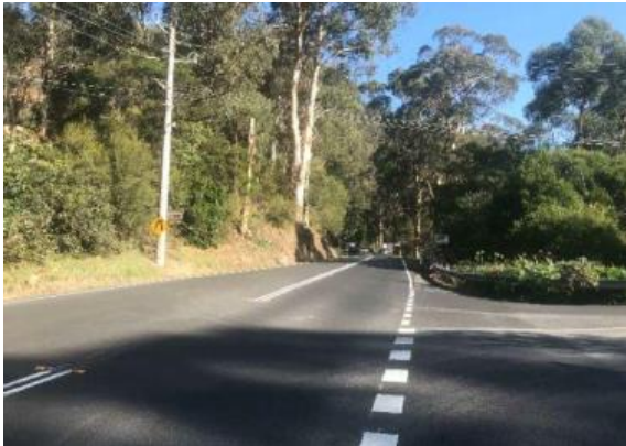
Figure 13-5 Warburton Highway & Mayer Bridge Intersection (facing west) Source: SALT 2019 TIA
