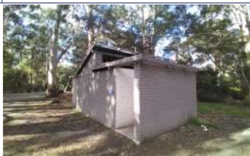
Dee Road toilet block
