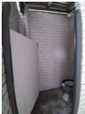
Dee Rd toilet block
