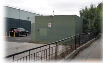
Rear entrance ramp to Churinga Shopping Centre
