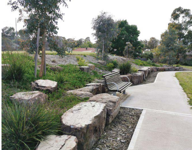
figure 5 Stone retaining wall and planted embankment
