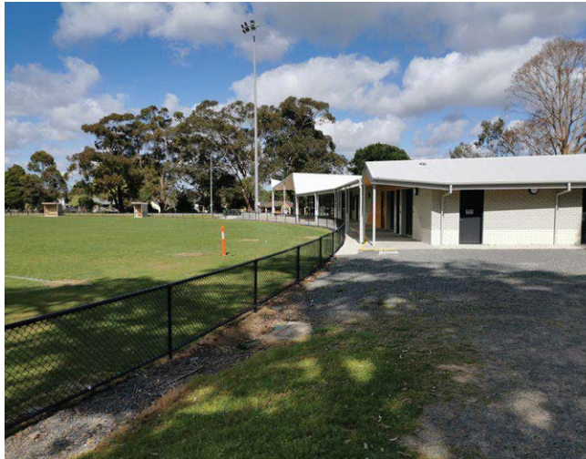
figure 6 Existing AFL Pavilion
