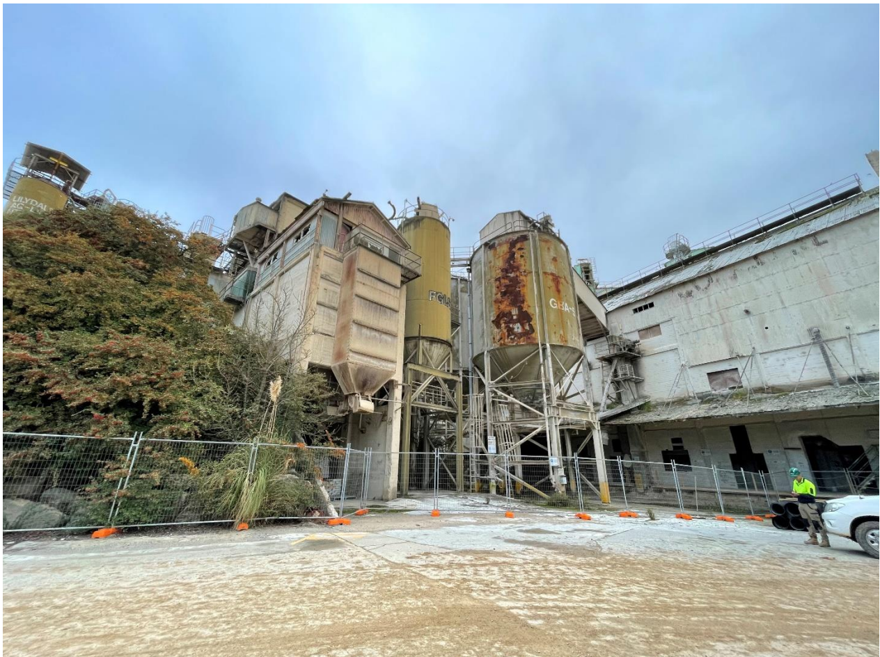
Remnant Quarry Processing Infrastructure
