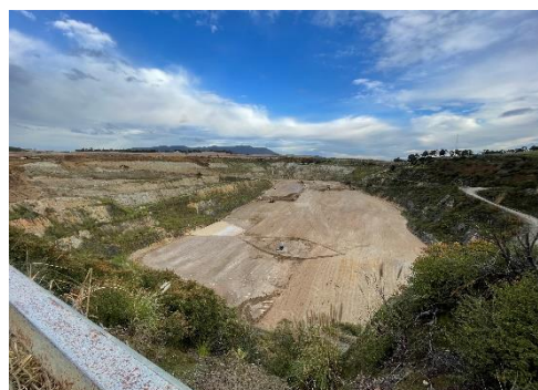
Existing Quarry Pit – Refilling in Progress
