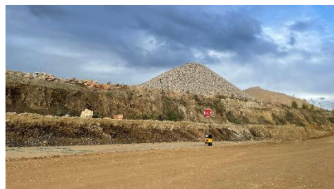
Existing Overburden Mounding – relocation
