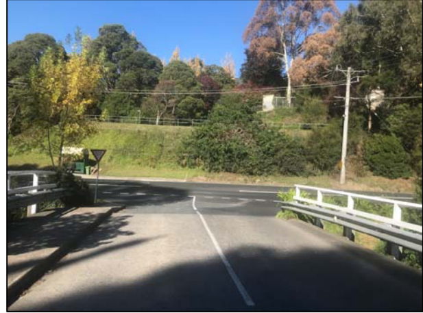
Figure 8 Mayer Bridge facing south
