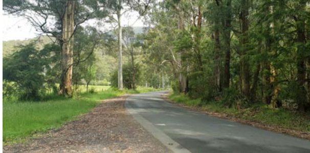
Figure 16 Warburton Highway, Wesburn
