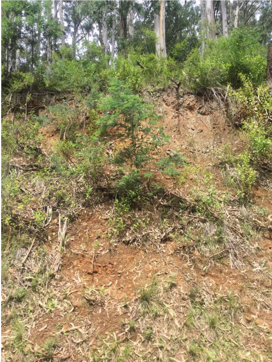
Photo 15 Steep road cutting in residual to extremely weathered siltstone
