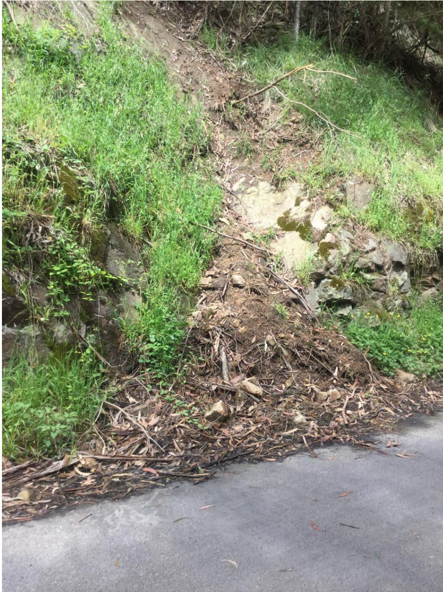
Photo 11 Recent debris material transported from above soil slopes down rock chute
