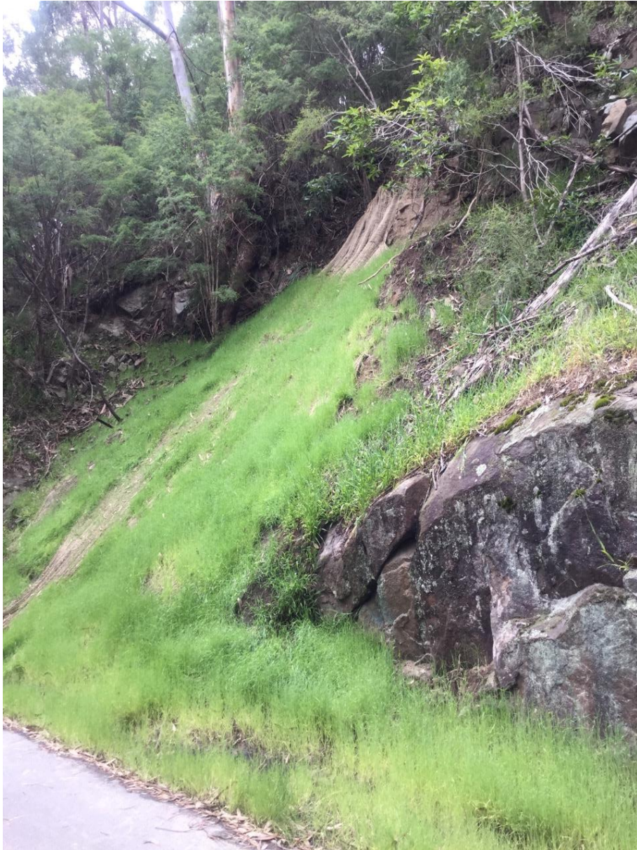
Photo 10 Back scarp of recent failure
