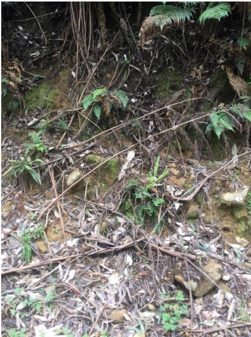
Photo 1 Typical weathered rhyodacite soil (2m high face)
