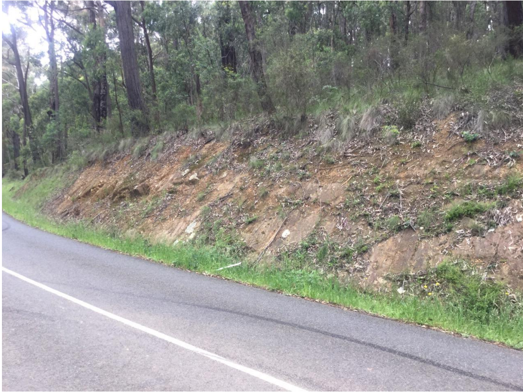
Photo 16 Road cutting showing thin soil cover (1-2 m) overlying siltstone rock
