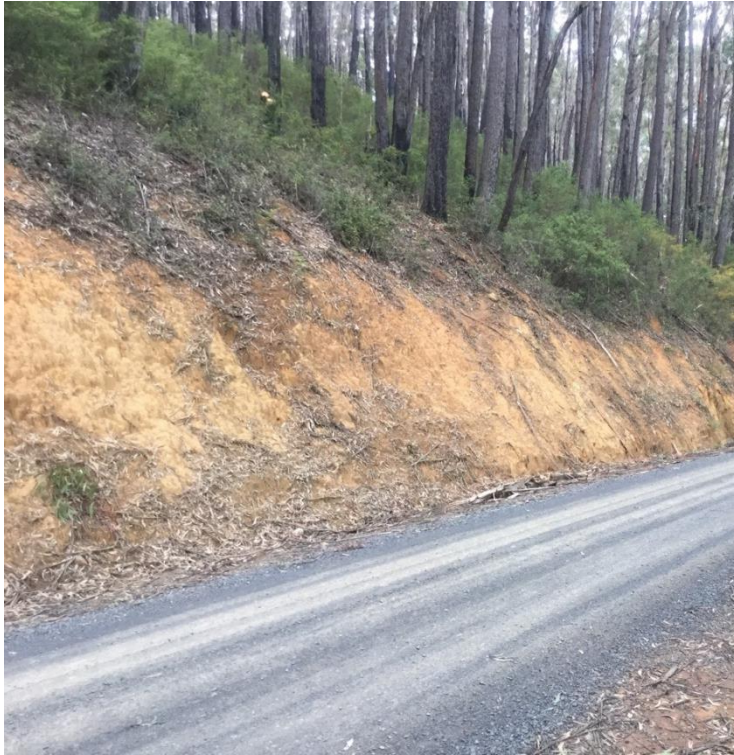
Photo 14 Road cutting in granitic soil standing at approximately 50-60 degrees
