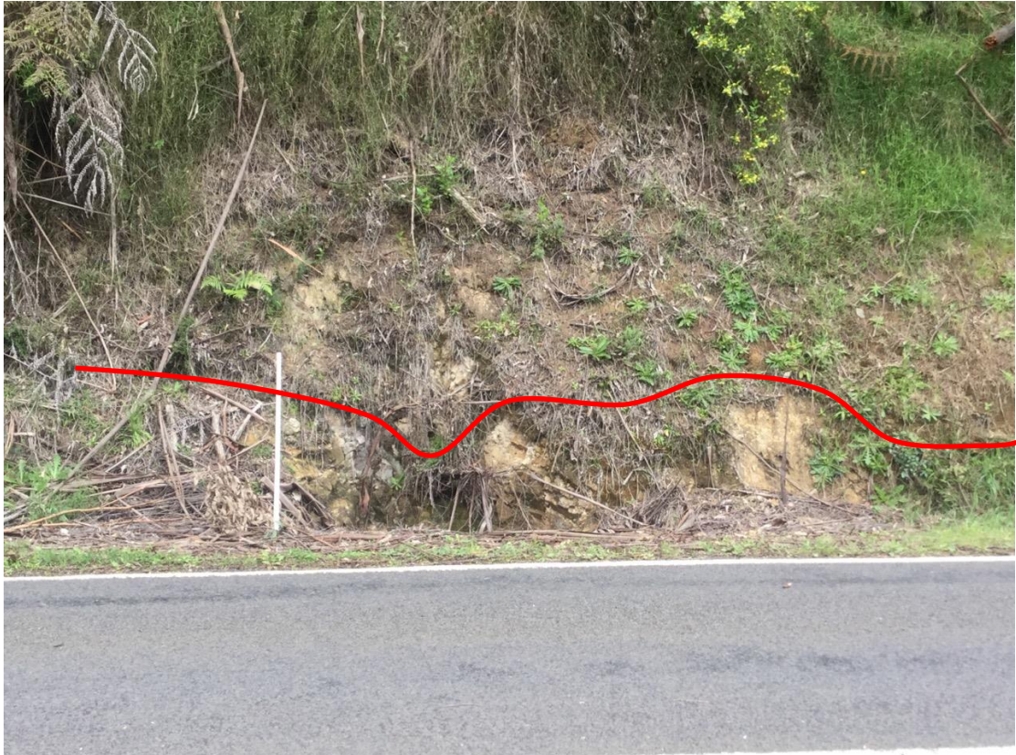
Photo 4 Interface between colluvium and rhyodacite rock. Colluvium consists of loose debris including rounded gravels and cobbles of rhyodacite. Outcrop in road cutting at the side of gully system
