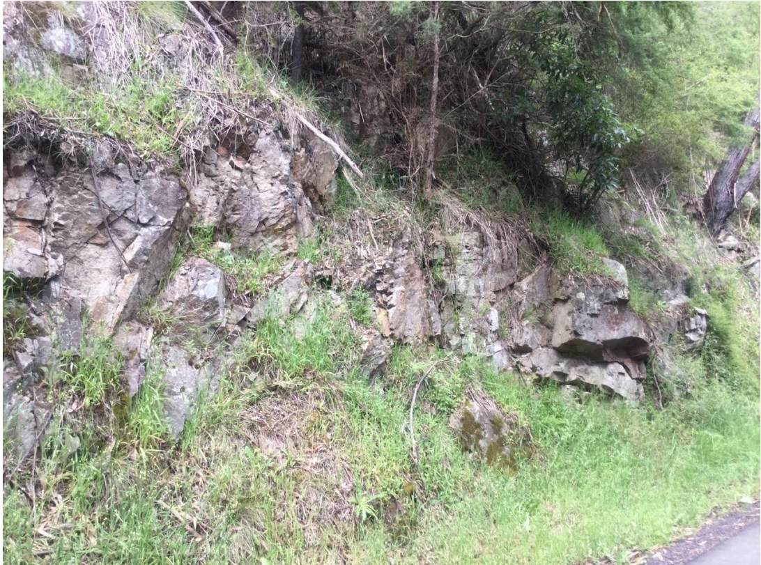
Photo 8 Rock mass observed in dyke cutting along Warburton rail trail
