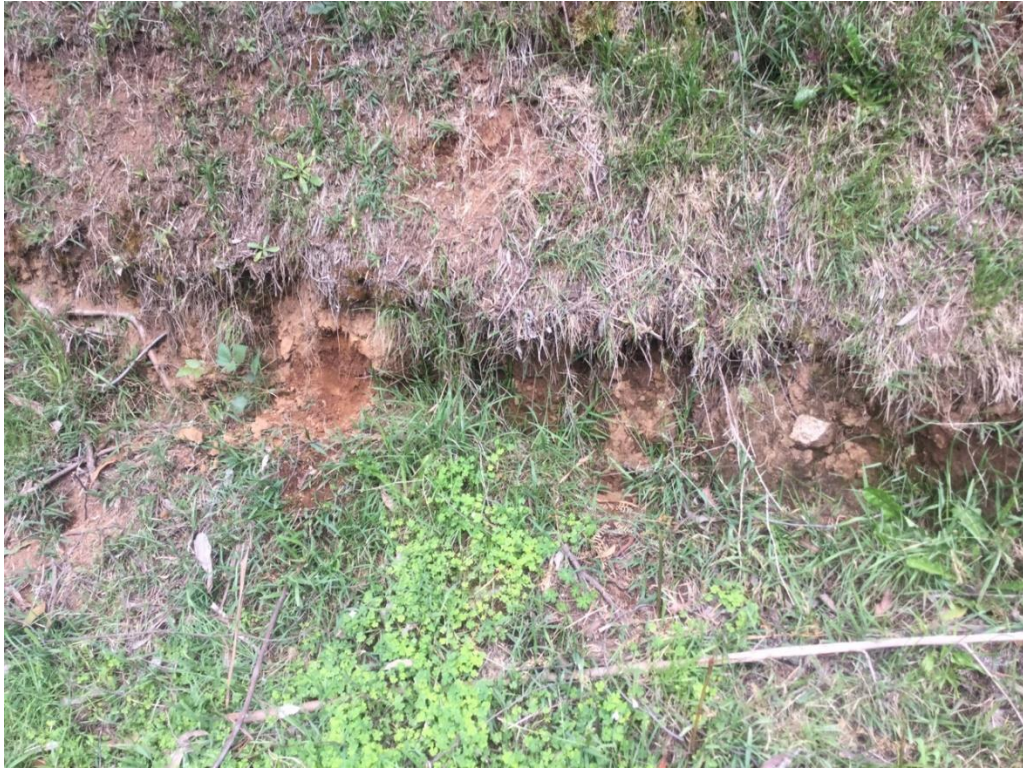
Photo 6 Unstable colluvium deposited within a gully which appears to have failed from over steepening of road cutting
