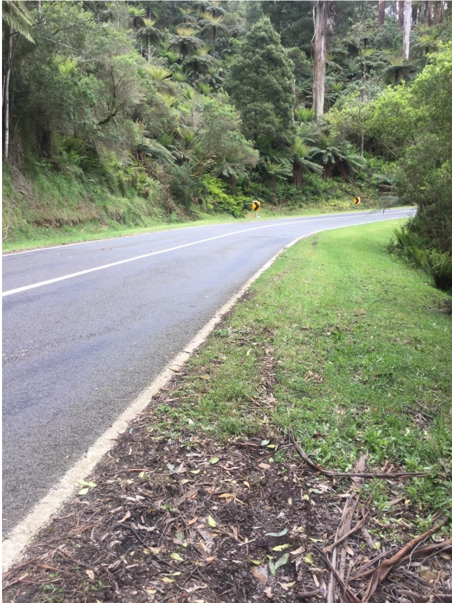
Photo 2 Colluvial deposit observed either side of channel slopes, underlying and down slope of the road. Tension cracking is observed in the road as well as slumping of the colluvial material downslope. Cleared/fallen trees within gully system that appear to be have been caused by the debris flow.
