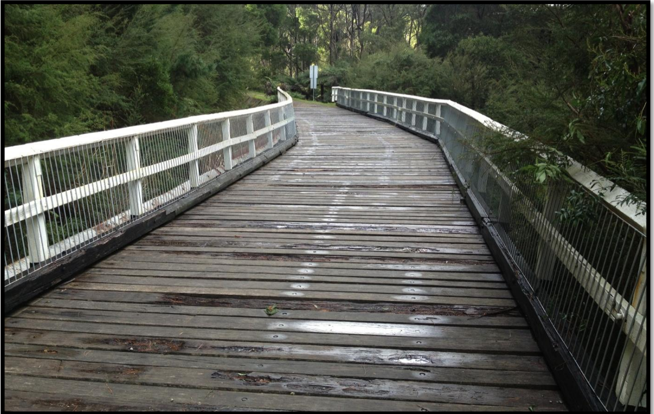
Figure 29. Bridge on the O'Shanassy Aqueduct
